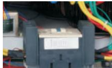
A.C.contactor: Using the best quality-85% silver point to make sure long life, meanwhile to make machine runs silently
